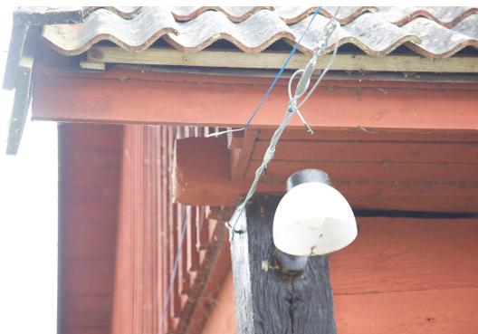
One end of the 70 meter long wire, with fiber
